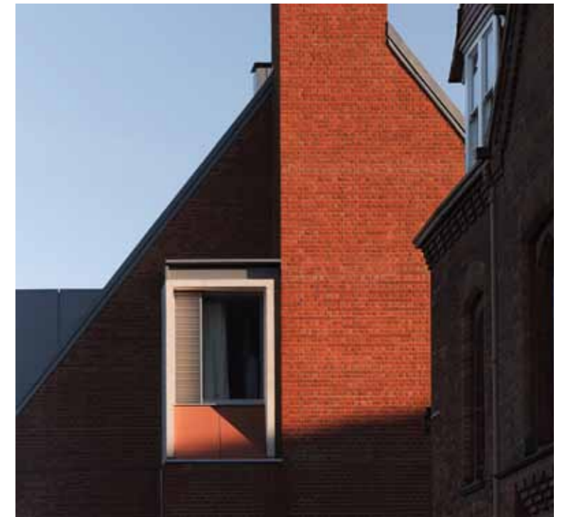
Above Gable end. Concrete frames the window ensemble and terracotta cladding. Left North-east elevation. Each bedroom has a fixed main window alongside a louvred panel in front of an insulated vent.
